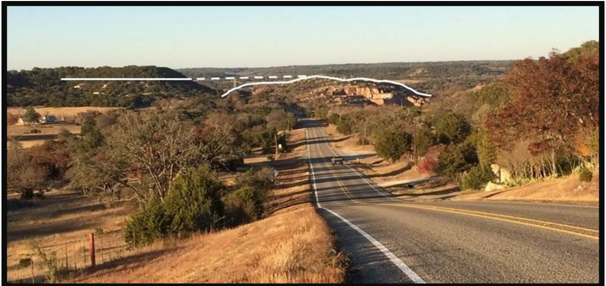
Image: Top of Bear Mountain (pre-Cambrian granite pluton) reaches upward to base of Edwards Limestone (horizontal white line); it represents an igneous spire standing more than 300' above the base of the Hensel Sandstone. Irregular convex-upward arch (white line) is Wichita Paleo Plain. (photo credit: Pete Rose)
