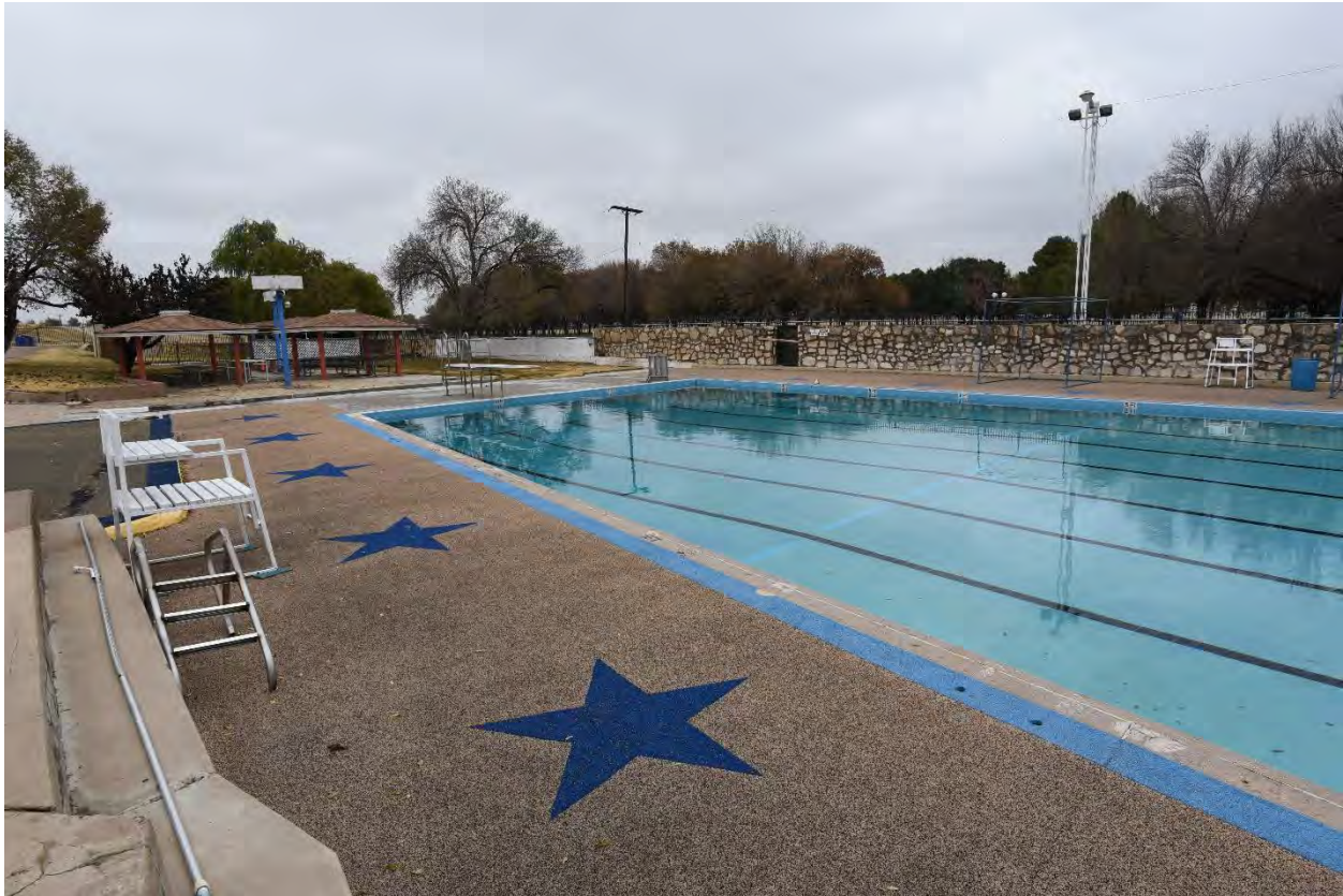
Figure 1. Looking northeast from the west/southwest side of the pool. The retaining wall is directly below the deck at the camera position.
