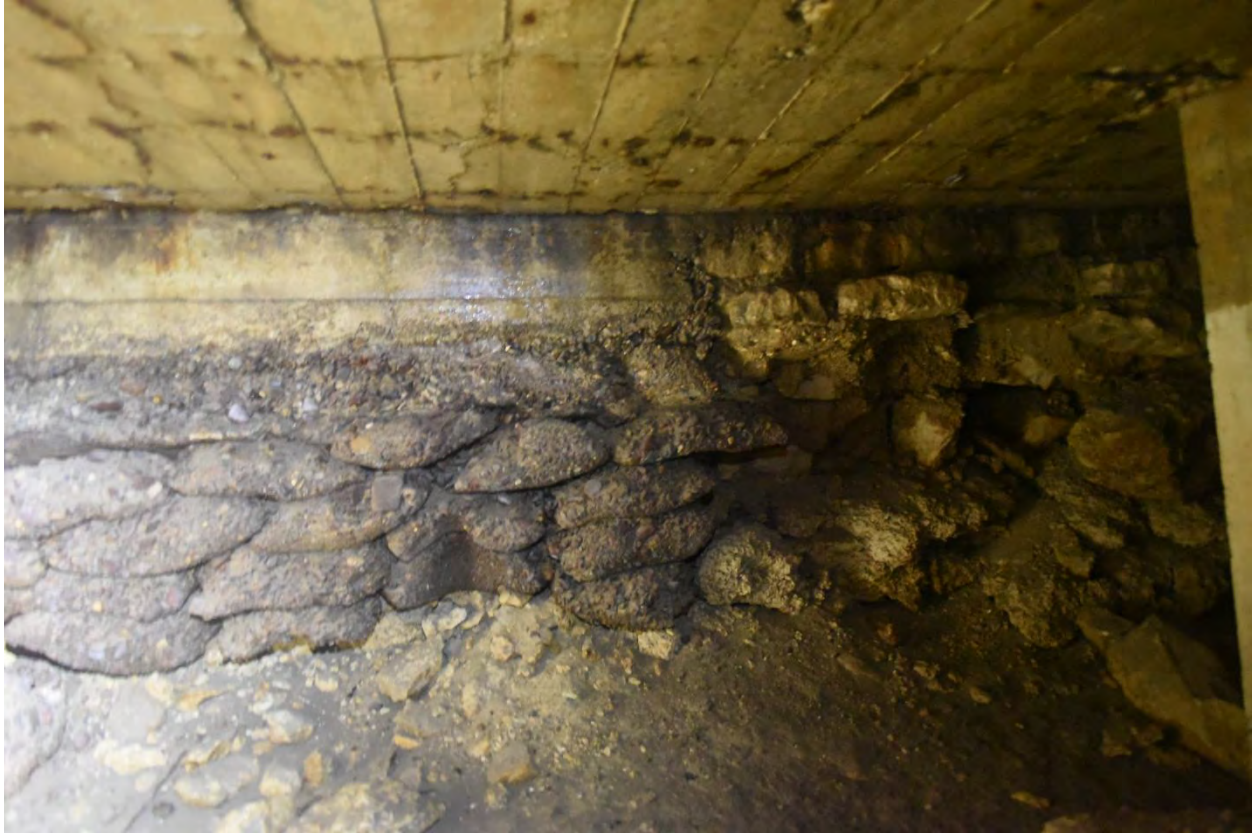
Figure 13. Wall repair using bagged materials.
